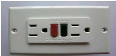
The GFCI is an inexpensive device which measures the difference in current levels going to and returning from a piece of electrical equipment. How does this device protect against shock?
