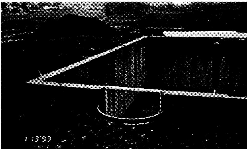
Figure 12. Completed Stemwall Foundation at the Eldersberg Site.
